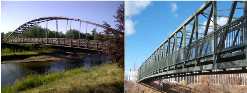
Figure 11: Examples of Pedestrian Bridges over the South Platte River Identifying Possible Pedestrian Bridge Structure Types
