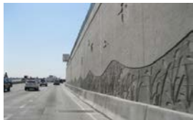
Alameda and I-25 wall treatments
