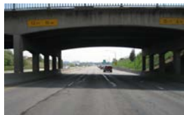
Existing Federal Boulevard Bridge over US 6
