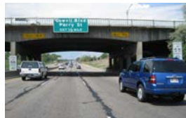
Westbound US 6 at the Federal Boulevard Bridge
