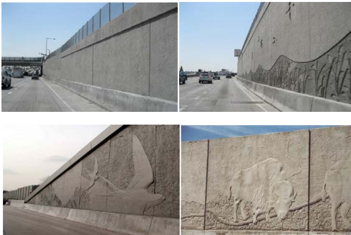
Figure 13: Different Retaining Wall Form Liners and Patterns
